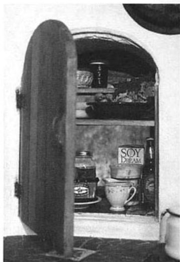
THICK WALLS ALLOW FOR A "COOL BOX" INSIDE THEM.
